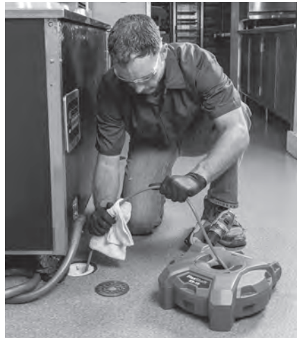
Figure 15 – Applying Lubricant to the Cable Sheath
