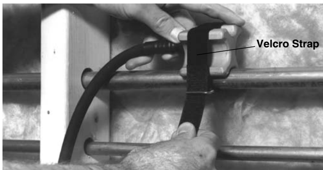
Figure 5 – Applying Freeze Head with Velcro Strap
