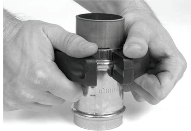
Figure 8 – Installing Press Ring Onto Fitting
