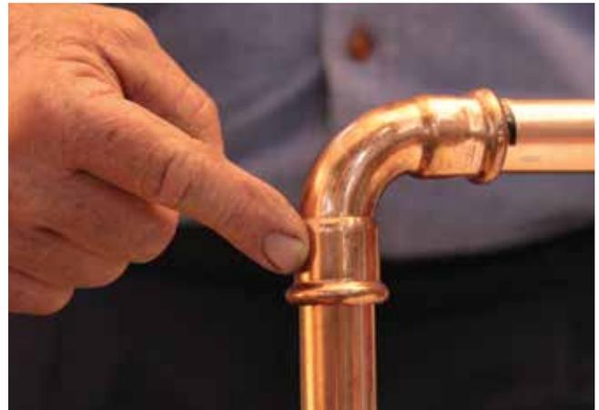
**9.** Visually inspect the fitting to ensure the press has been completed. The KemPress® tool will flash if the fitting did not press correctly. If this occurs a new fitting and tube section is required. At the end of the project visually inspect each fitting to ensure none have been missed.
