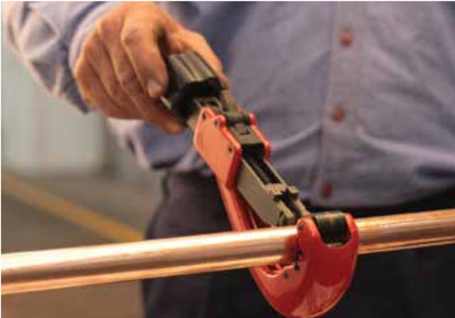
**1.** Cut copper tube to length using a pipe cutter.
