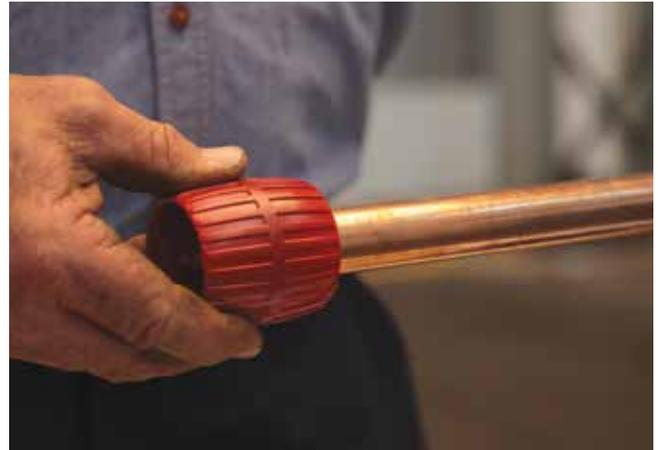
**2.** Deburr carefully the end of the tube on the inside to minimize turbulence and pressure loss according to the relevant plumbing code and on the outside to avoid damaging the O-ring.
