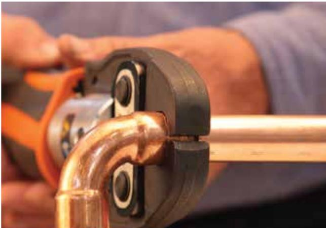
**8.** Initiate the pressing job by pressing the start button. The automatic pressing process creates a tight connection.
