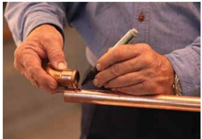
**4.** Mark the insertion depth by lining up the fitting side by side with the tube and mark the tube. When the fitting is inserted onto the tube the outer edge of the fitting must line up with the marking. For correct insertion depths see the table below.
